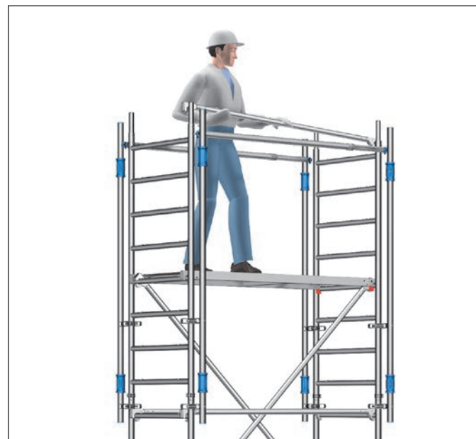
Fig. 6: Safe fitting of the guardrails with AGR
