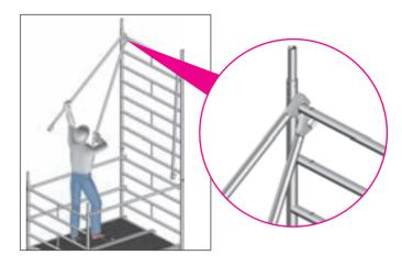
During dismantling of an intermediate or working platform, first remove the topmost rear guardrails from the level underneath them. This is done with the aid of a rear guardrail installed at knee level.
