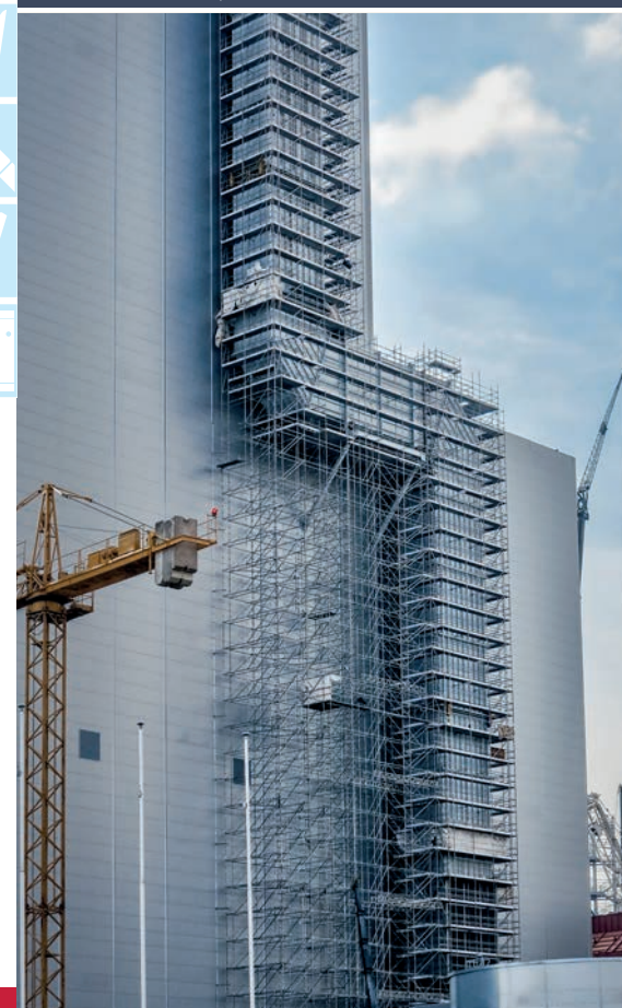
Wood-free work scaffolding at power station
