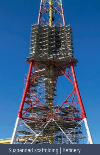
Suspended scaffolding | Refinery
