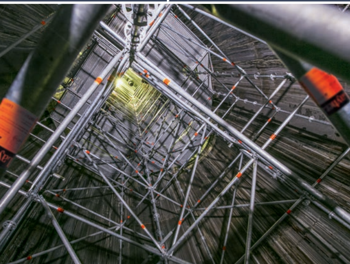
Allround LW in boiler of a paper factory
