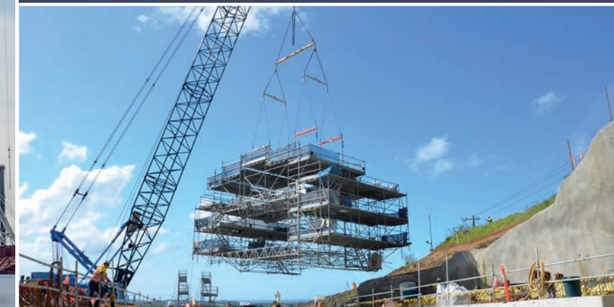
Crane-movable tunnel scaffolding | Tunnel repair
