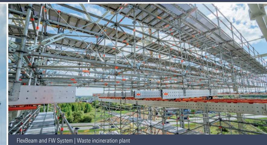
FlexBeam and FW System | Waste incineration plant
