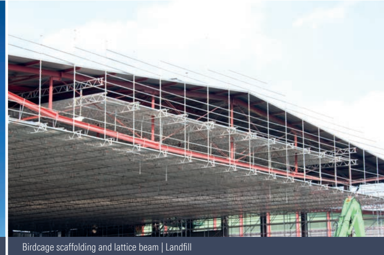
Birdcage scaffolding and lattice beam | Landfill
