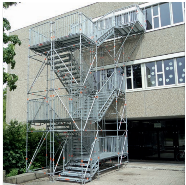
Adaptation of the entry and exit levels at the stairway bottom or top area using equalising stairways with different heights.
